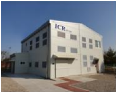
Ex Test Building
