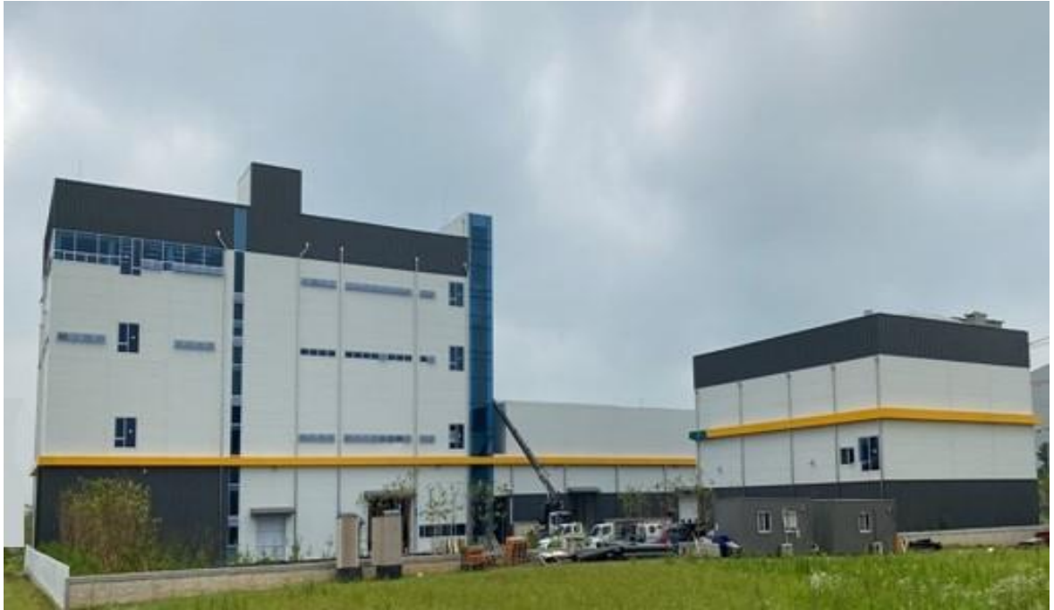
<View of ICR Pyeongtaek Battery Testing Center>
